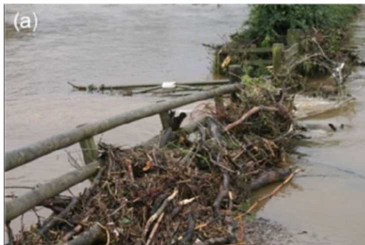
Figure 1 – image sources from Prof Andy Russell (2015) [4] which illustrated the blockage risk due to debris capture that fences within the floodplain may pose.
